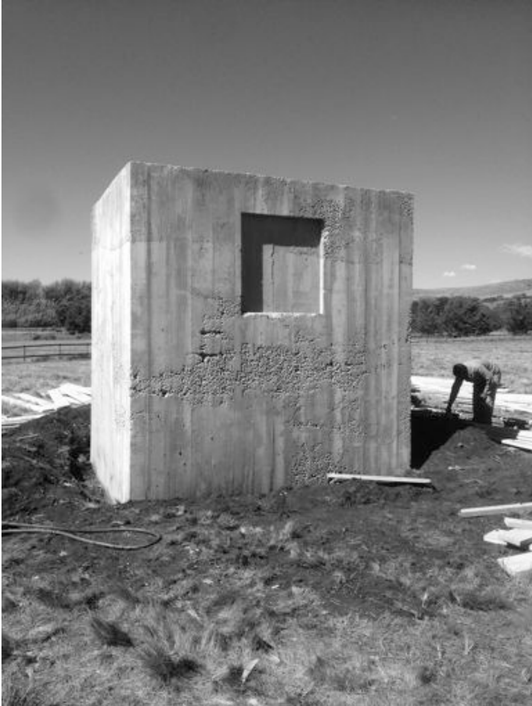
Cell after shutter removal.
